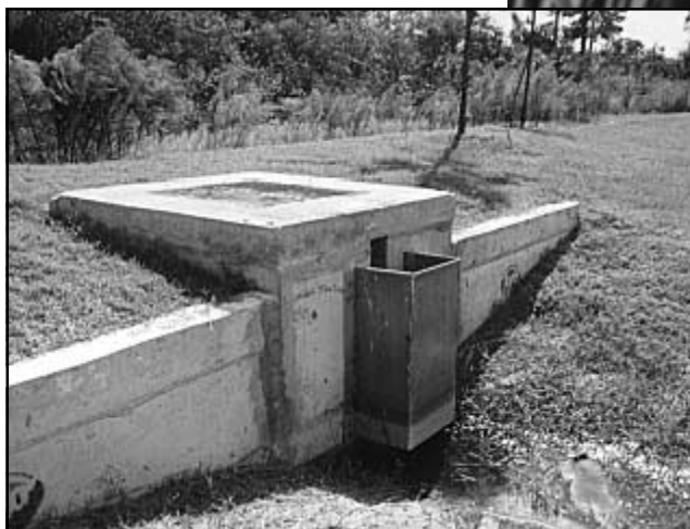
▲ Outflow Control Structure
