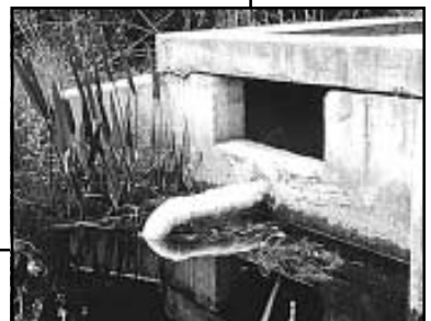
▲ Wet detention pond outfall structure.
