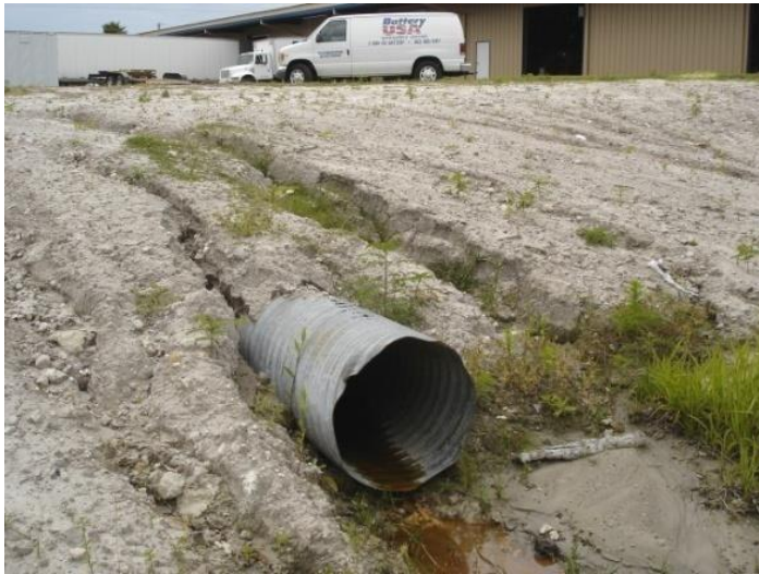
Example of Bank Erosion
