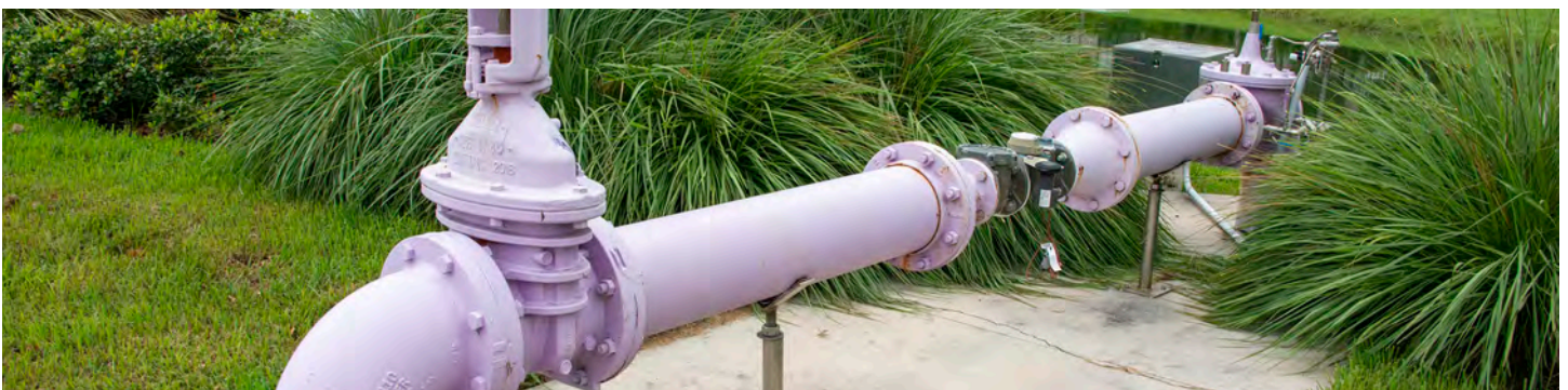
Top: A great blue heron admires a stormwater pond at Stoneybrook Golf and Country Club, Sarasota FL; Bottom: Reclaimed irrigation water from purple pipes may be high in nutrients | David Shafer .
